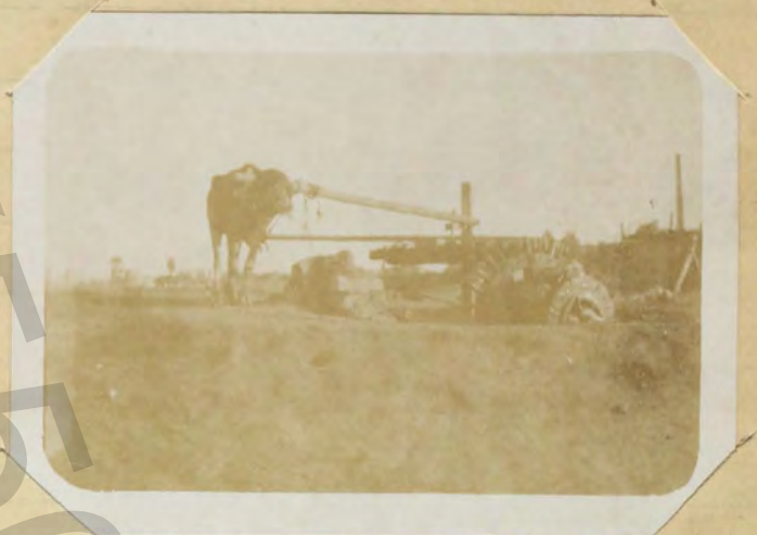
Water wheel for irrigation
